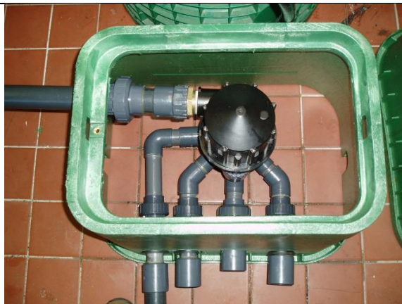
Example of a 4 zone pipe network using a 4 outlet indexing valve
