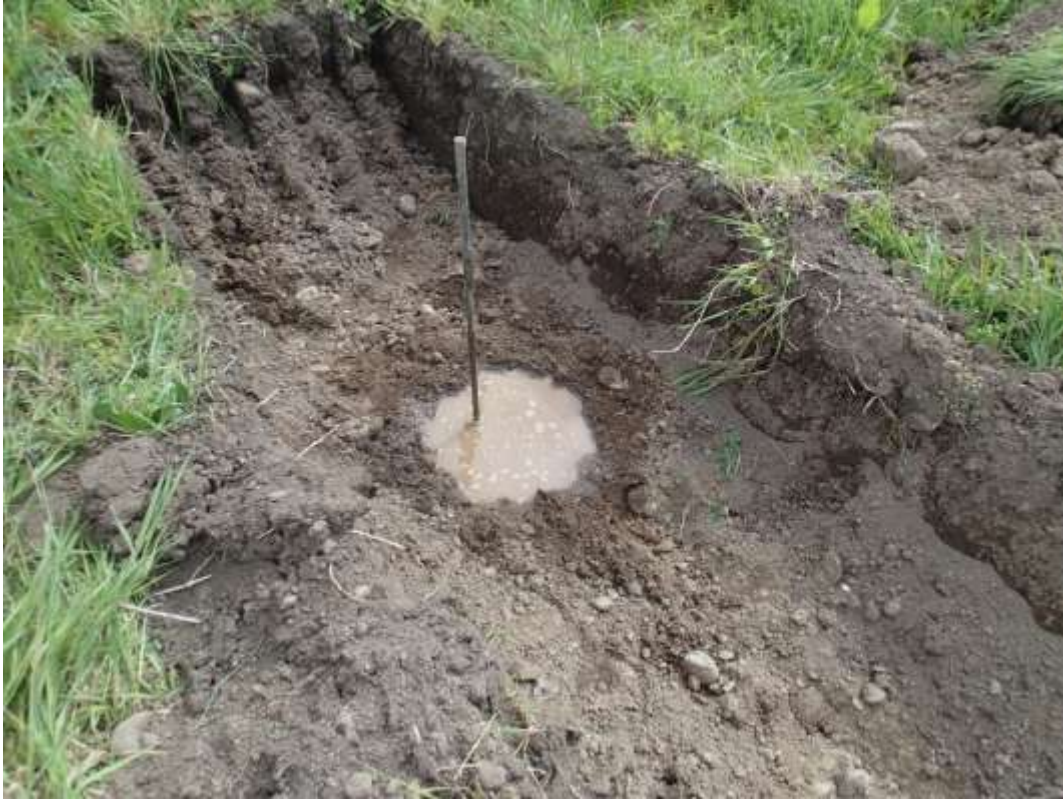
Plate 5: Water falling on morning of Tuesday 12 th May 2015 in ‘T’ test hole number 2.
