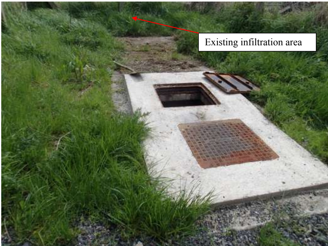
Plate 12: The existing septic tank system on the site, which must be decommissioned as part of the proposed development.
