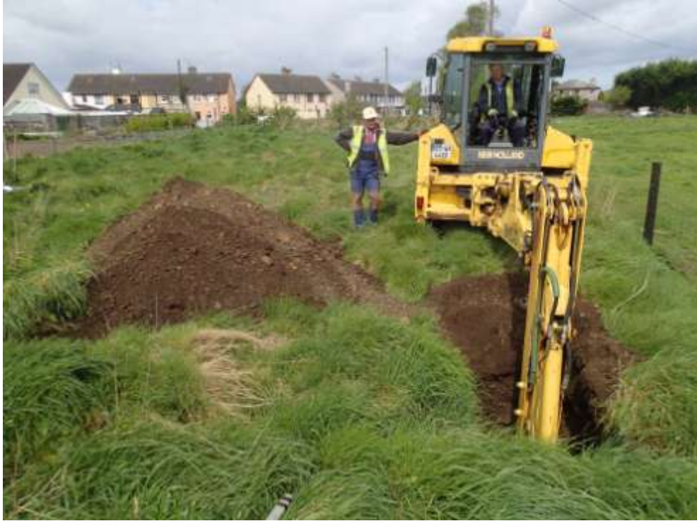
Plate 1: View of the site from the south, while excavating the test hole. See the well drained appearance of the land around the site. The holes were dug at the edge of the footprint of where the proposed polishing filter area will be located.
